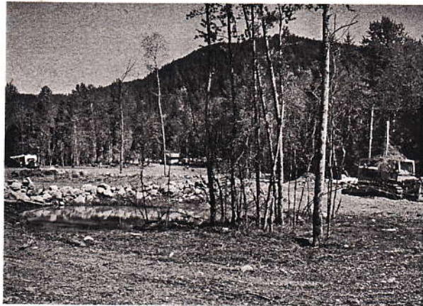
An example of the McDougal Brothers' destruction of forest habitat along scenic Highway 242.
